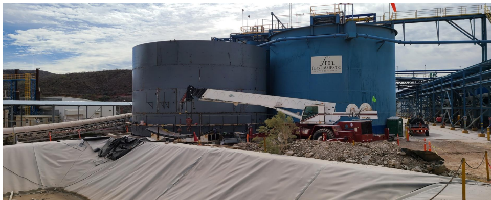
Figure 15 – Leach Tank #6 construction progress, January 2022
