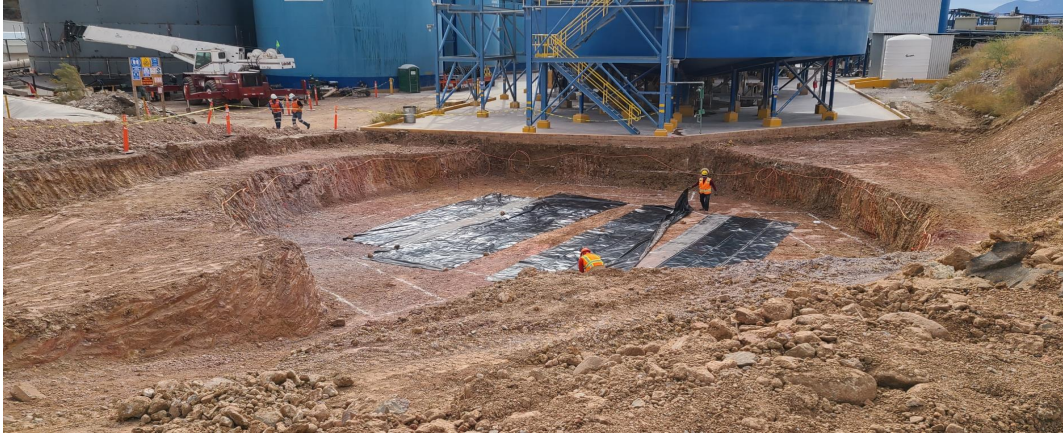
Figure 16 – CCD4 thickener earthworks progress, January 2022
