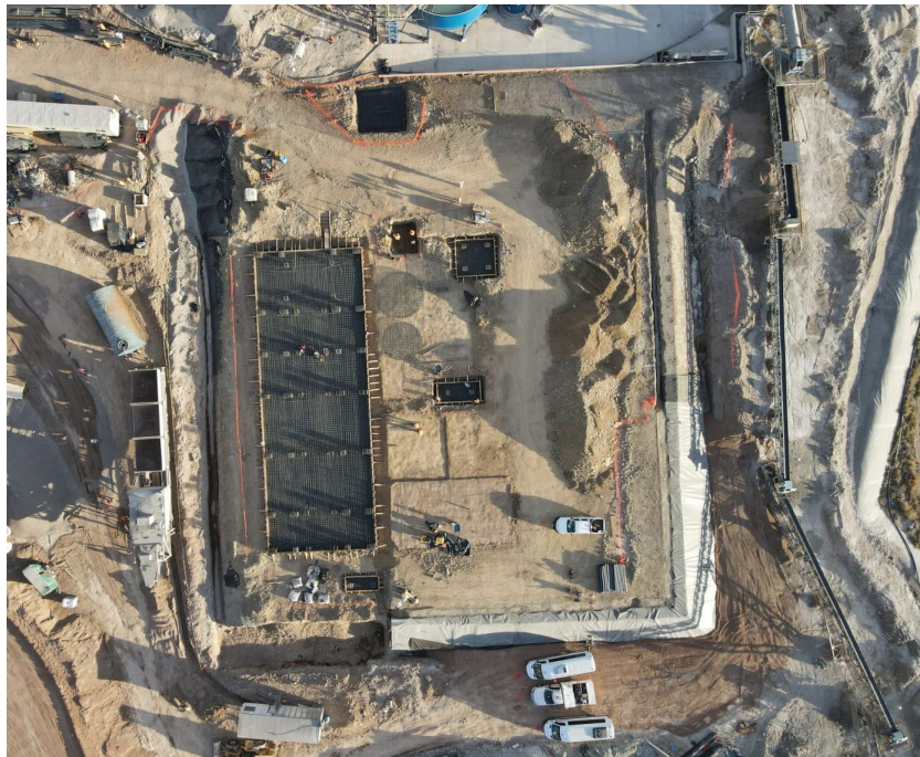
Figure 17 – Fast filter press circuit construction progress, January 2022
